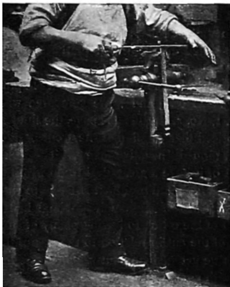
FIG. 2.—Position when filing.
