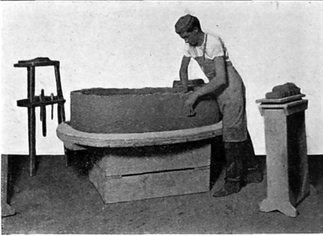
FIG. 145.—Working finger courses and filling in.
