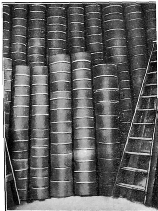
FIG. 114.—Saggars in position in oven.
