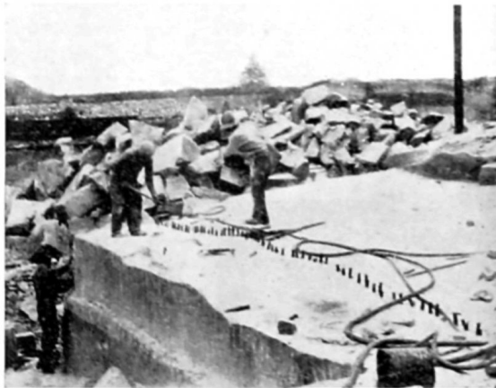
FIG. 7.—USE OF PLUGS-AND-FEATHERS IN QUARRYING. (By courtesy of "The Stone Trades Journal.")
