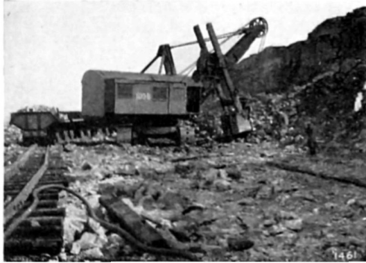
FIG. 3.—MECHANICAL NAVVY. (By courtesy of Ruston-Bucyrus Ltd.)
