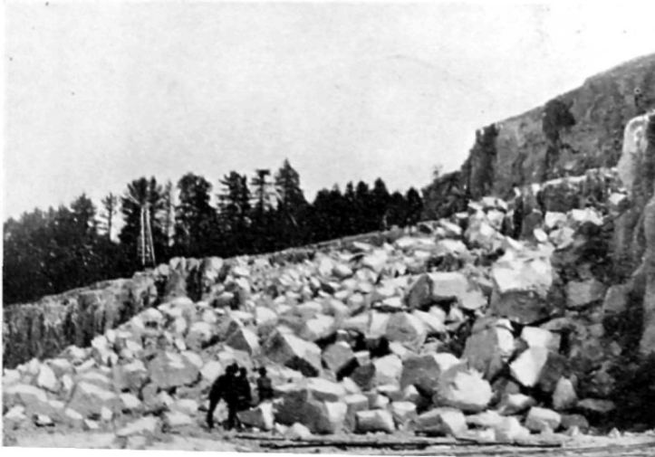
FIG. 10.—EFFECT OF EXPLOSION BY LIQUID OXYGEN. (By courtesy of Liquid Oxygen Explosives Ltd.)
