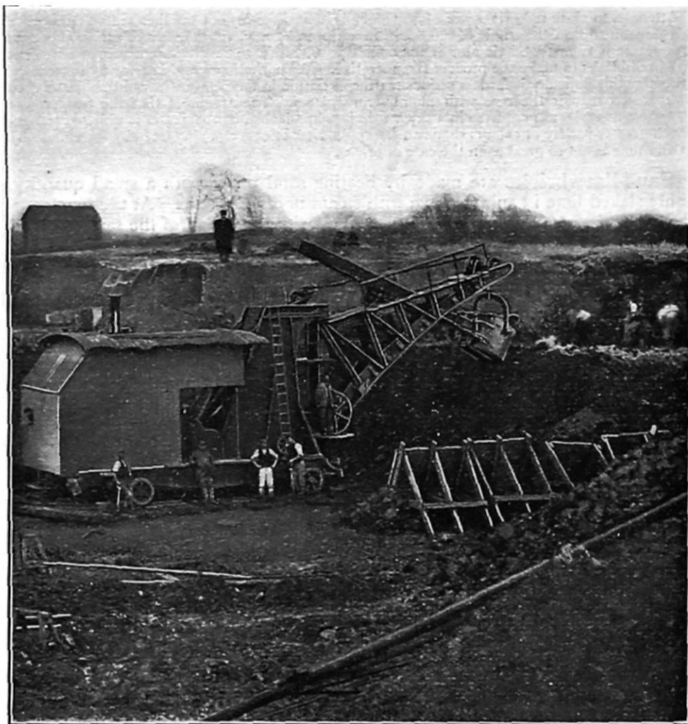
FIG. 1.—Steam Navy Digging Clay.
