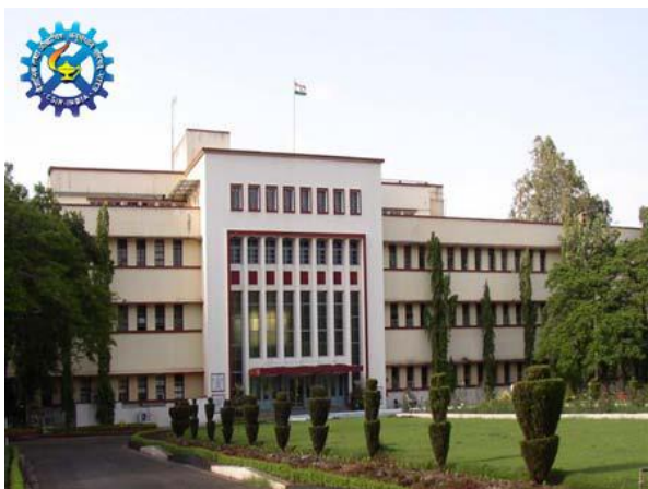
CSIR-NATIONAL CHEMICAL LABORATORY, PUNE
