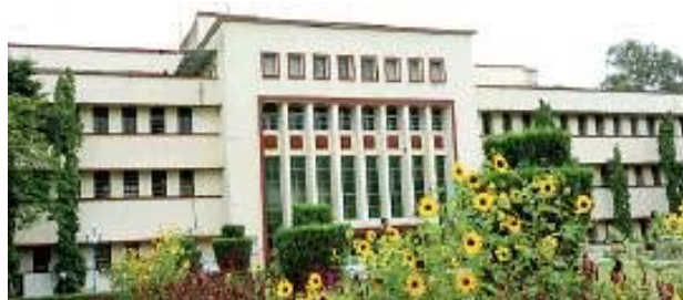
The Pashan facility where the break happened
