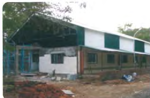
Lab Block progressing towards completion
