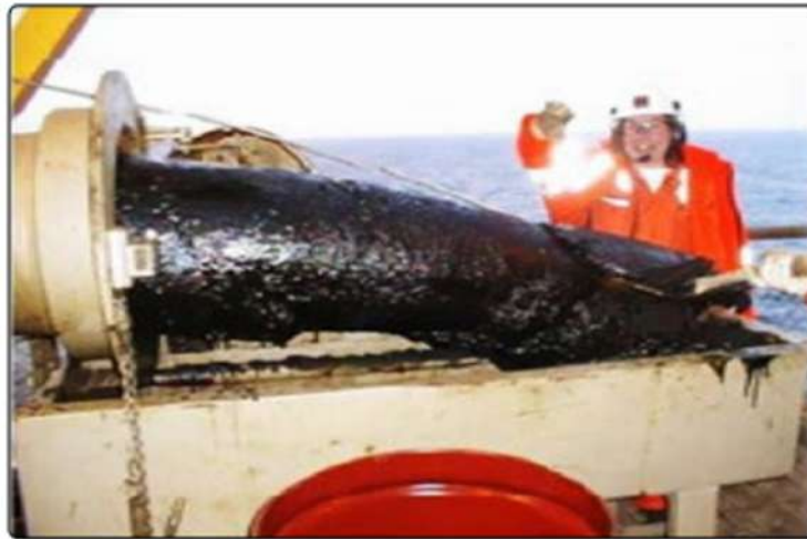
Figure 1.2 Blocked petroleum pipeline during shutdown period. This figure is reprinted from [25].
