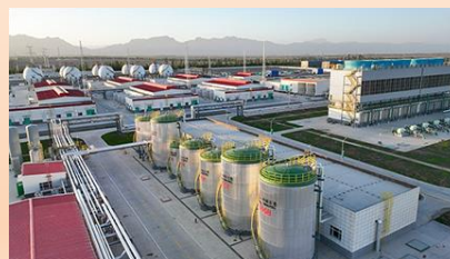
Aerial view of 20 KTPA photovoltaic Green Hydrogen Pilot Project—Sinopec's Kuqa facility, Xinjiang, China
